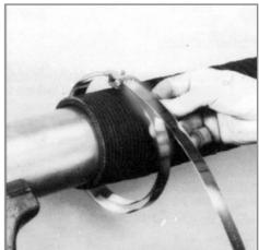
Follow same steps to double wrap for added radial compression. Bend end of band under buckle.
